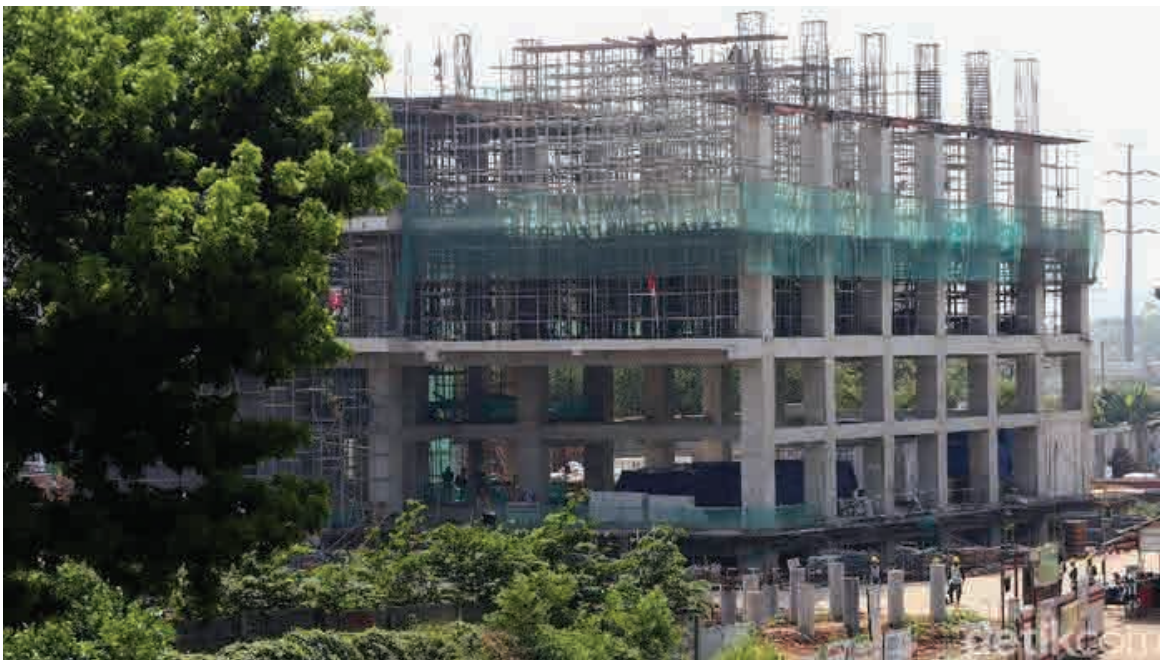
Gedung OCC + Admint Building
